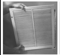
First remove your old grille by removing the screws. It may need to be pried off with a screwdriver if it is sticking to the wall paint.
