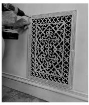
Install grille with the screws provided, then cover the screw heads with the vinyl tabs.
